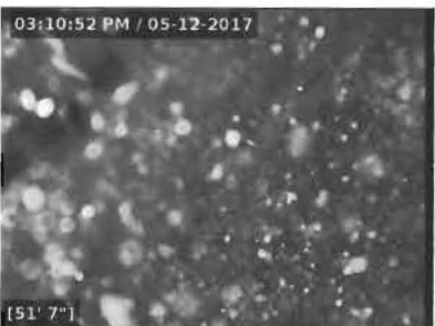
5/12/2017 3:10:53 PM front line entering tank, high liquid level due to backup from clogged backline
