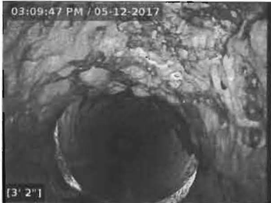
5/12/2017 3:09:47 PM change from cast iron to PVC front line
