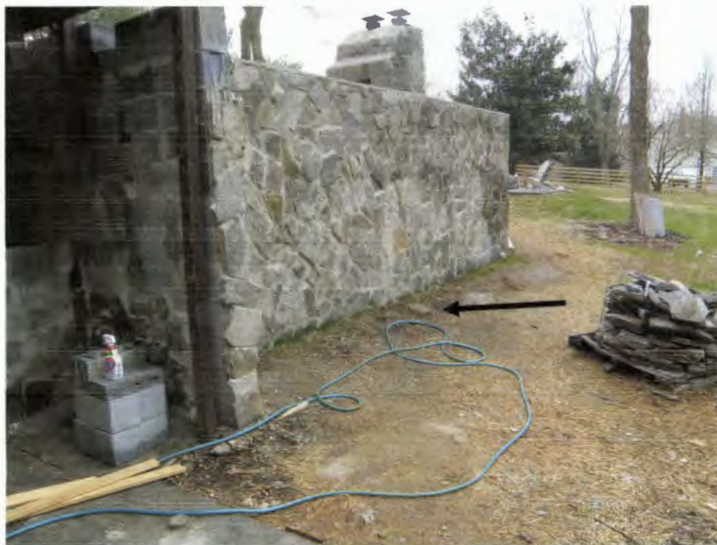
Photo 1 – Retaining wall, with cleanout at bottom of wall (Arrow)
