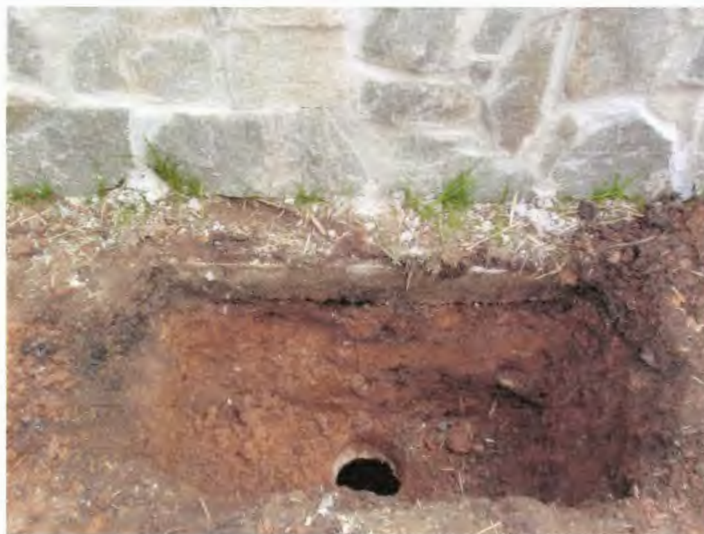
Photo 2 – Test pit at septic tank cleanout.
