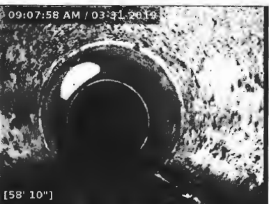
3/31/2019 9:07:59 AM Y joint in the front line
