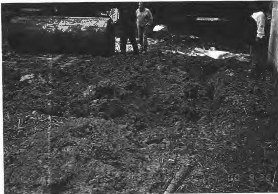
4. View of the removed UST next to the excavation pit.
