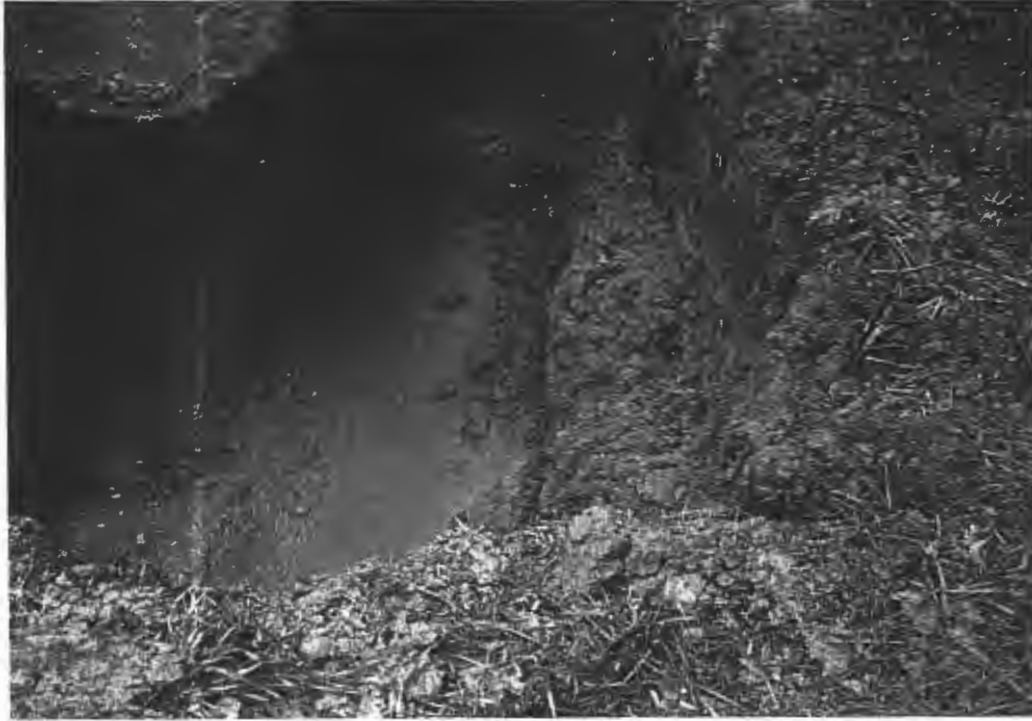
3. The UST excavation pit after removal of tank.
