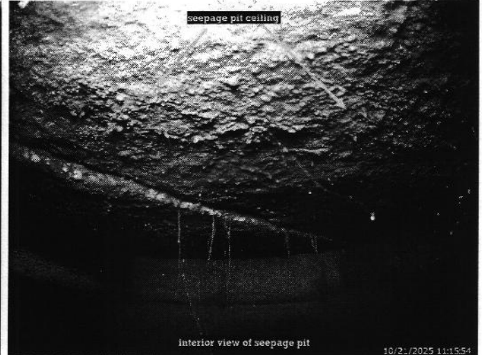
The seepage pit appears to be intact and functioning as intended at the time of the inspection.
