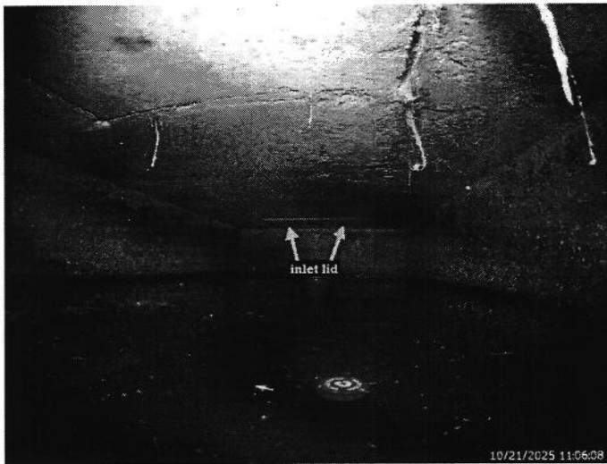
Concrete Inlet lid appears to be fully intact and working as intended at the time of the evaluation.
