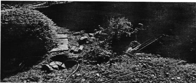
There are several plantings in the vicinity of the septic system, specifically the septic tank.
