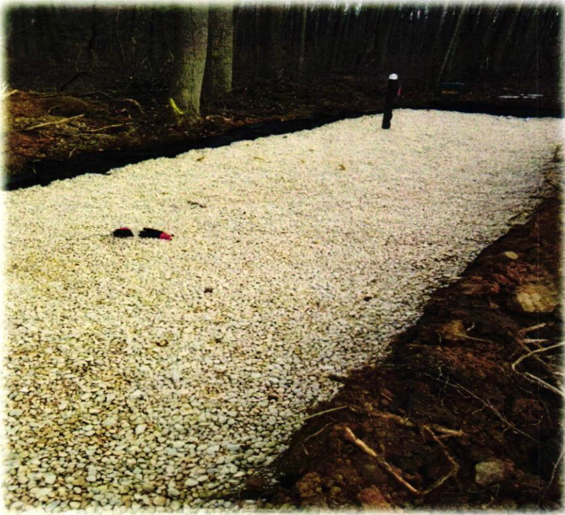
12470 Petrillo Drive – Washed river gravel LPD bed being installed with first of two obs. Pipes. –kmw 12/13/2017
