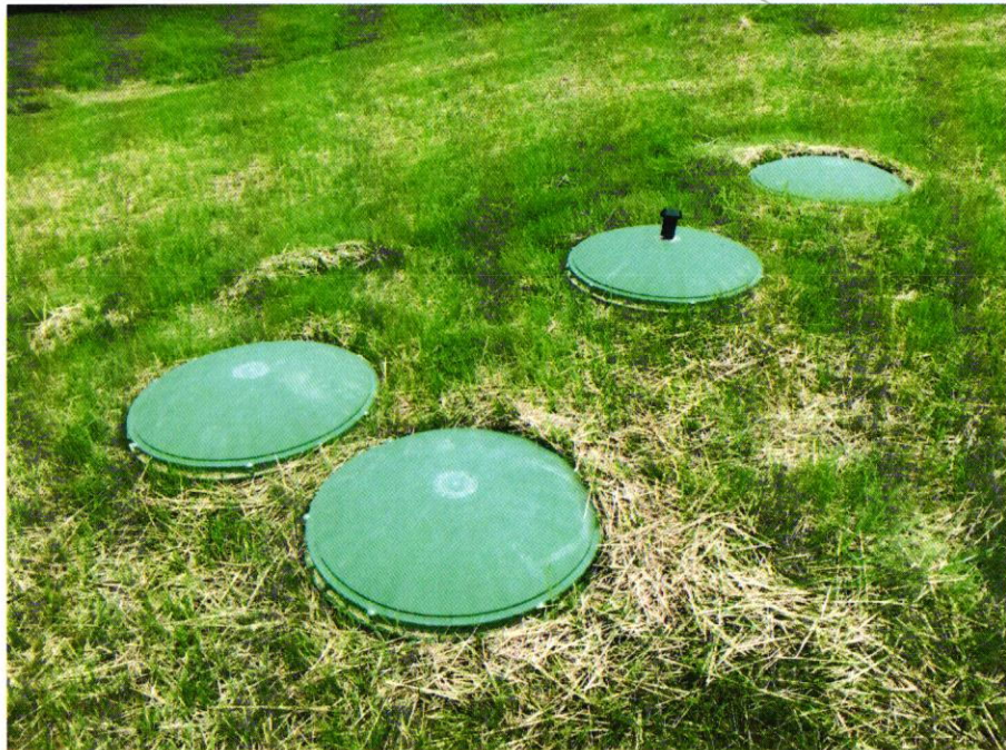
Grading around the septic tank
