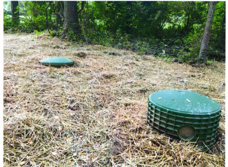
Grading around the pump tank
