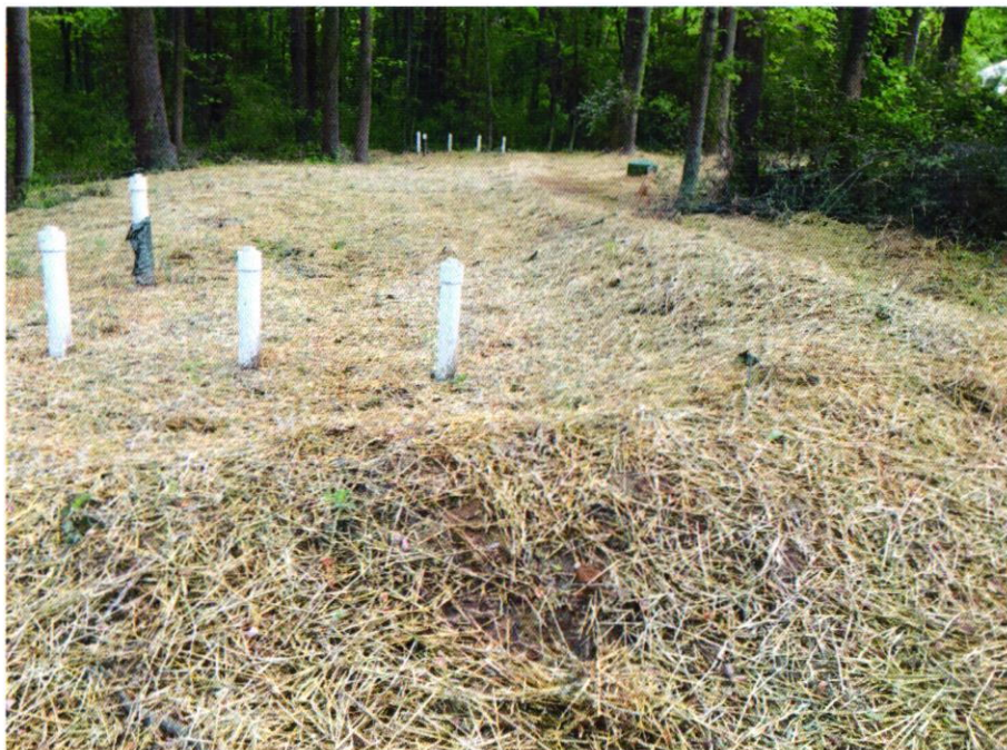
View of the berm from the N end
