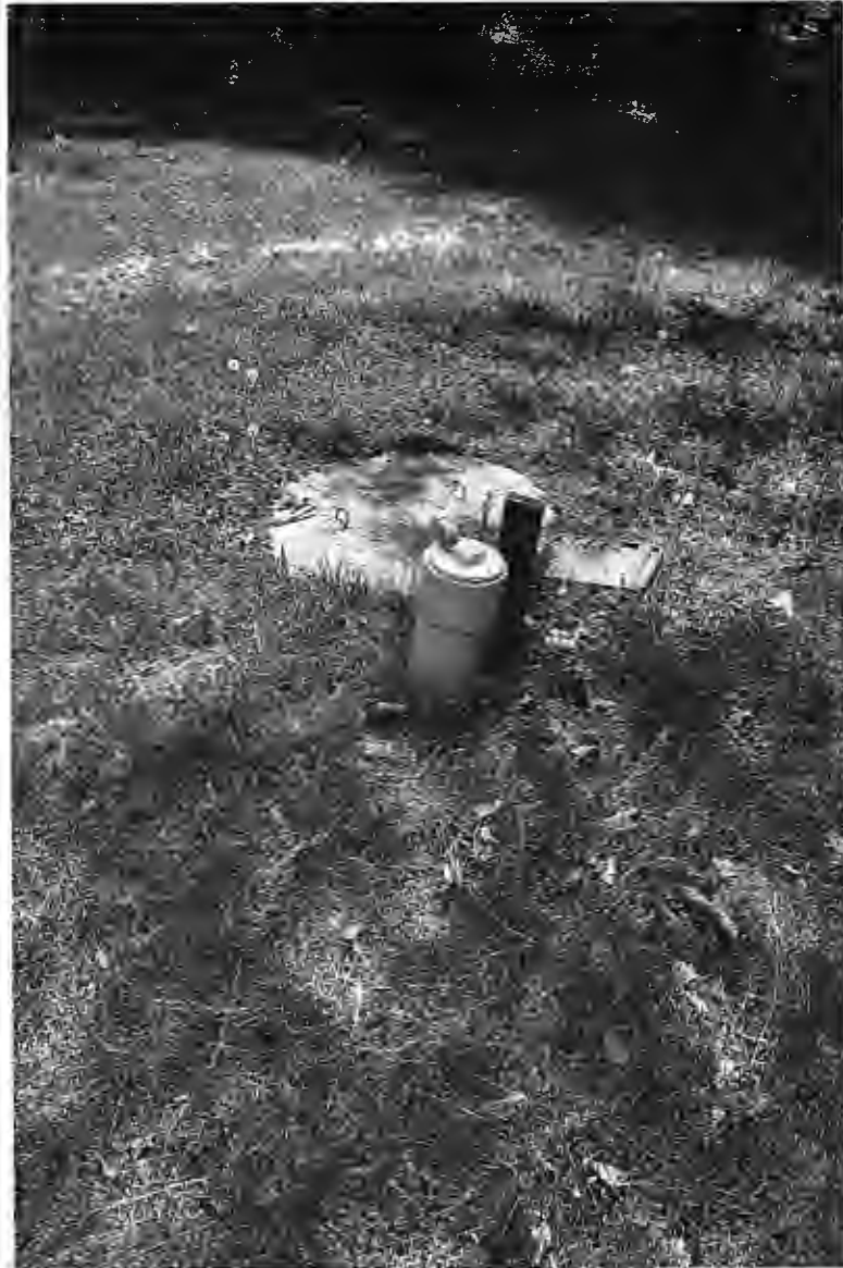
Ex. Pump Tank Site Visit to 4/30/2024
