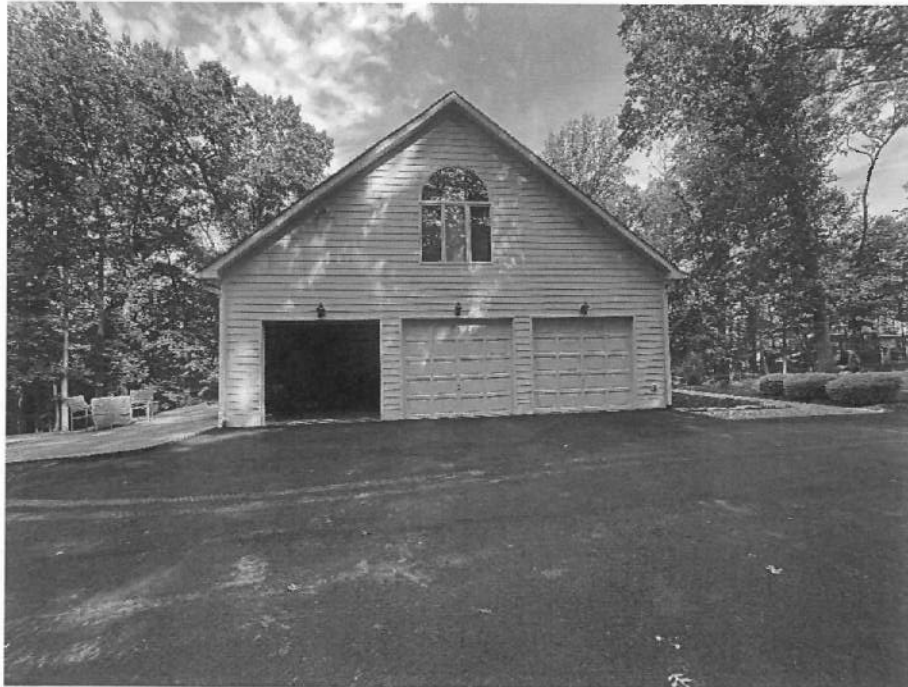
Photograph 4 - Left-side elevation of residence.
