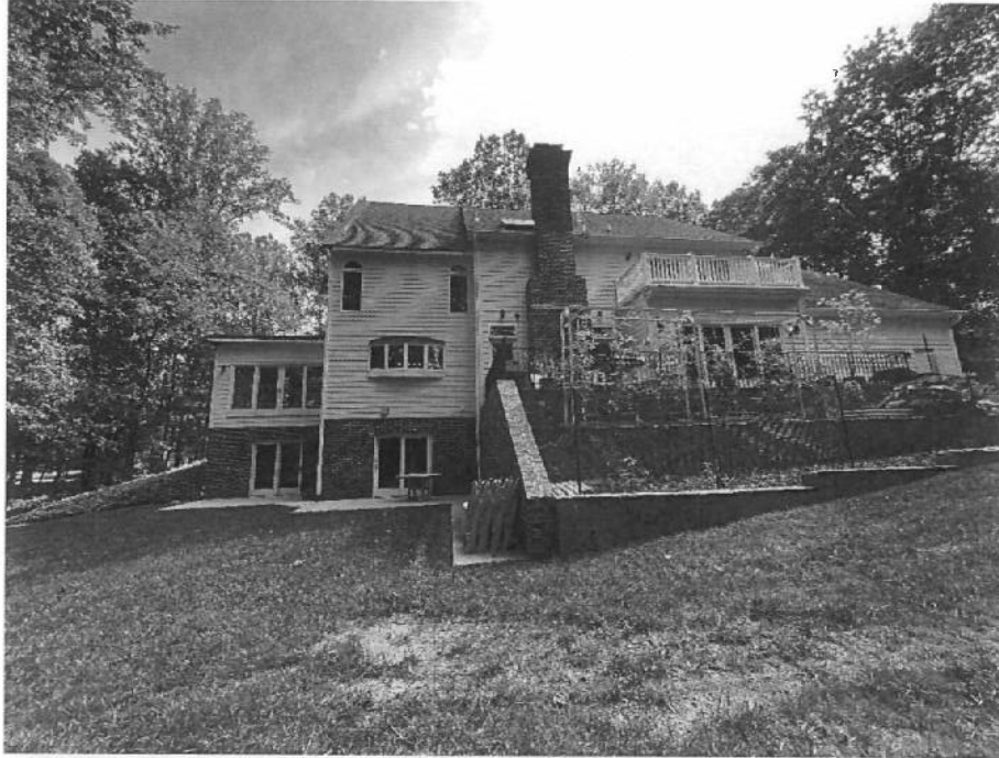
Photograph 3 - Rear elevation of residence.
