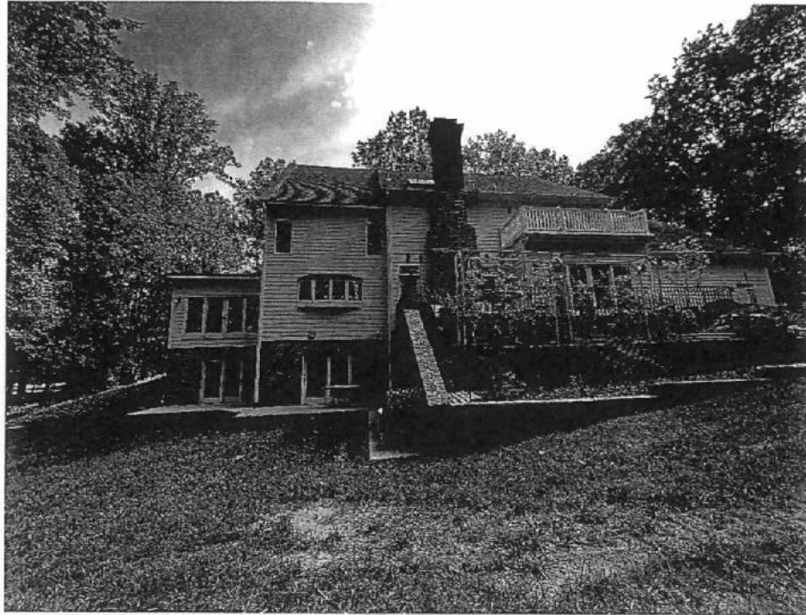
Photograph 3 - Rear elevation of residence.
