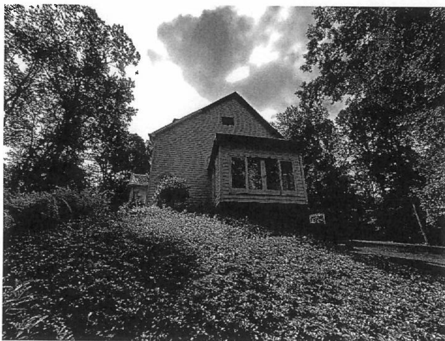
Photograph 2 - Right-side elevation of residence.
