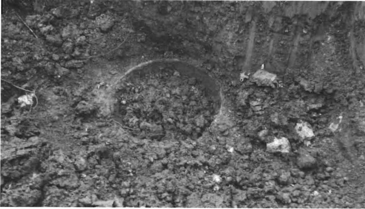
8690 Pine Road – Picture showing exposed well that appears to be sealed. 12/8/2015
