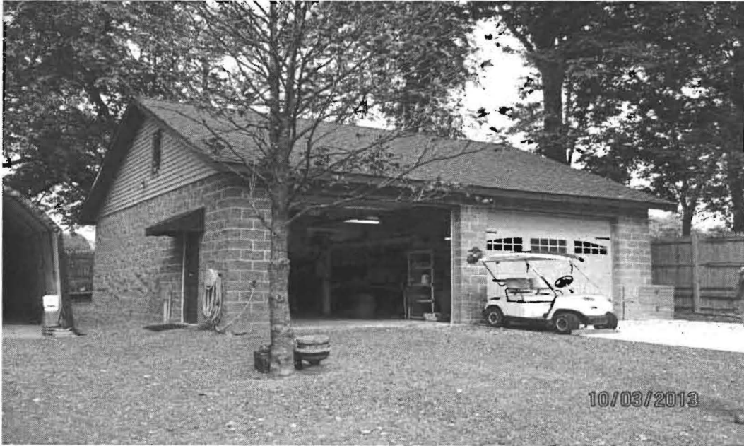
Detached 32x34 two car garage with rear 6x18 shed roof for storage.
