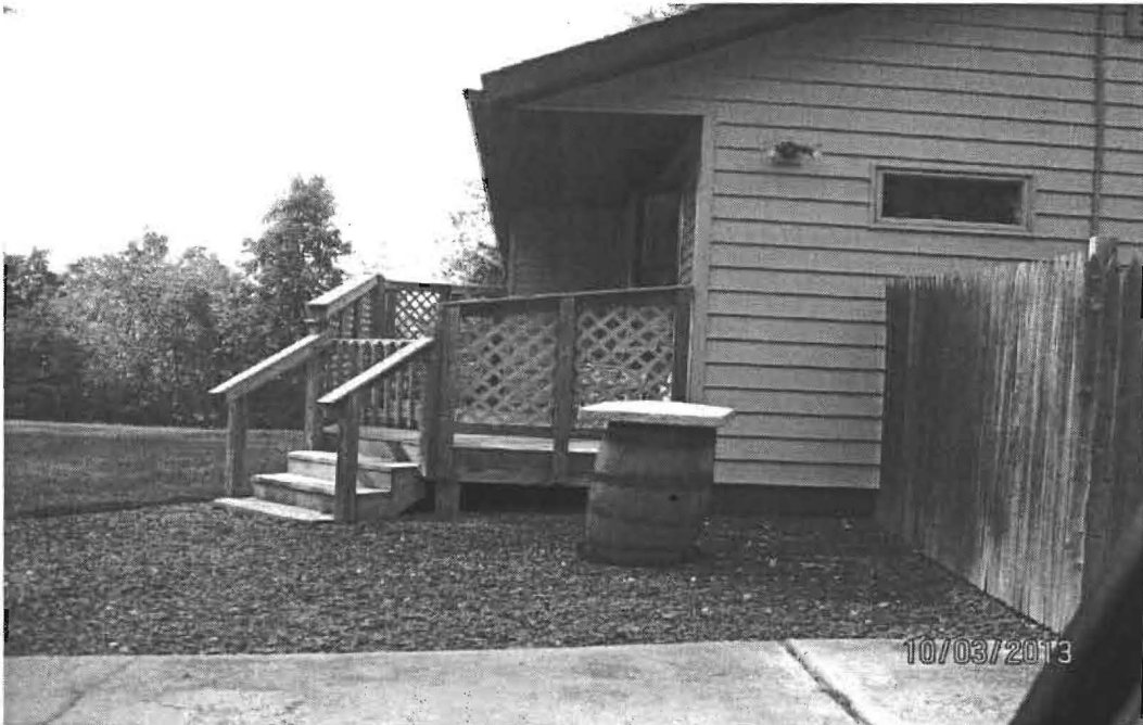
An 8x17 front entrance deck.
