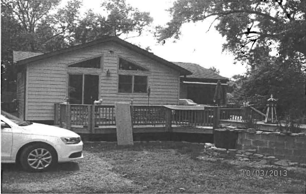
A rear 14x26 addition with wrap around deck.
