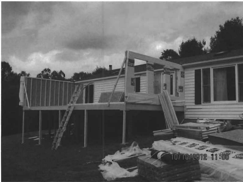
14' x 32' (approx.) addition viewed from right rear
