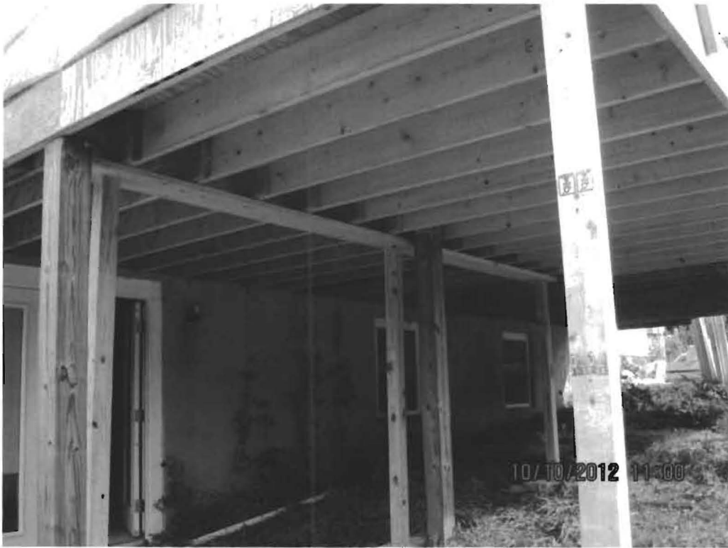
Underside of addition, beams not yet in place
