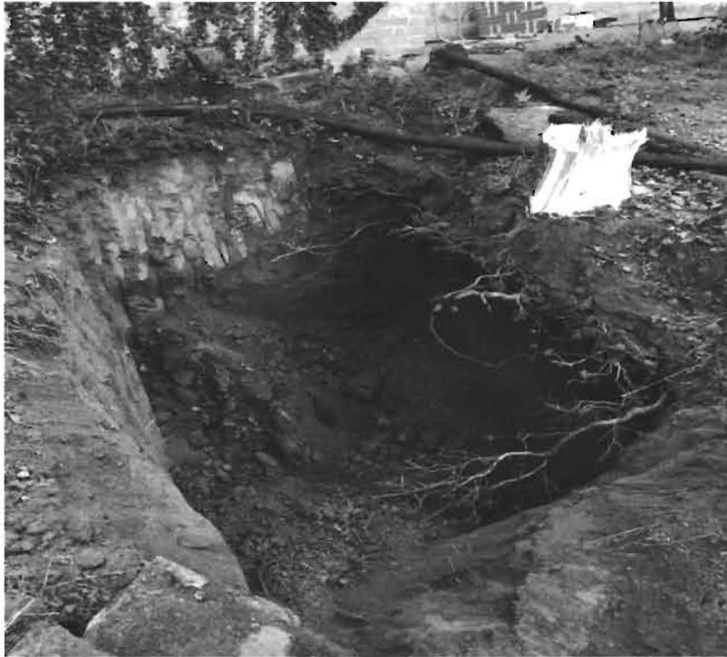
Photograph 3 Bottom of the diesel UST following removal
