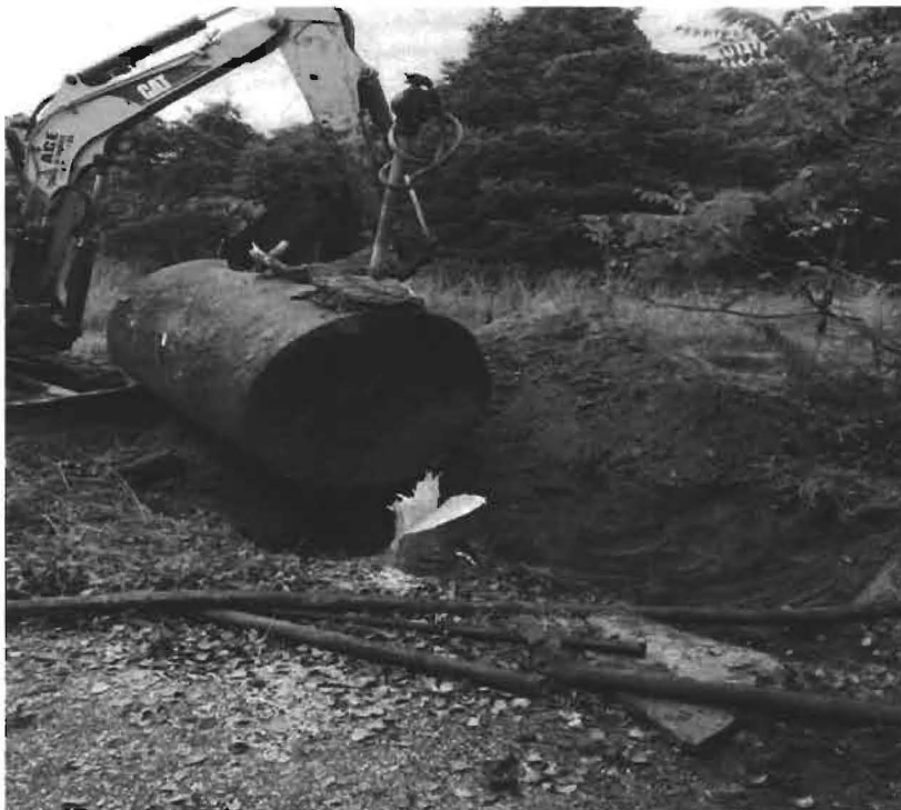
Photograph 2 Diesel UST being removed from the ground
