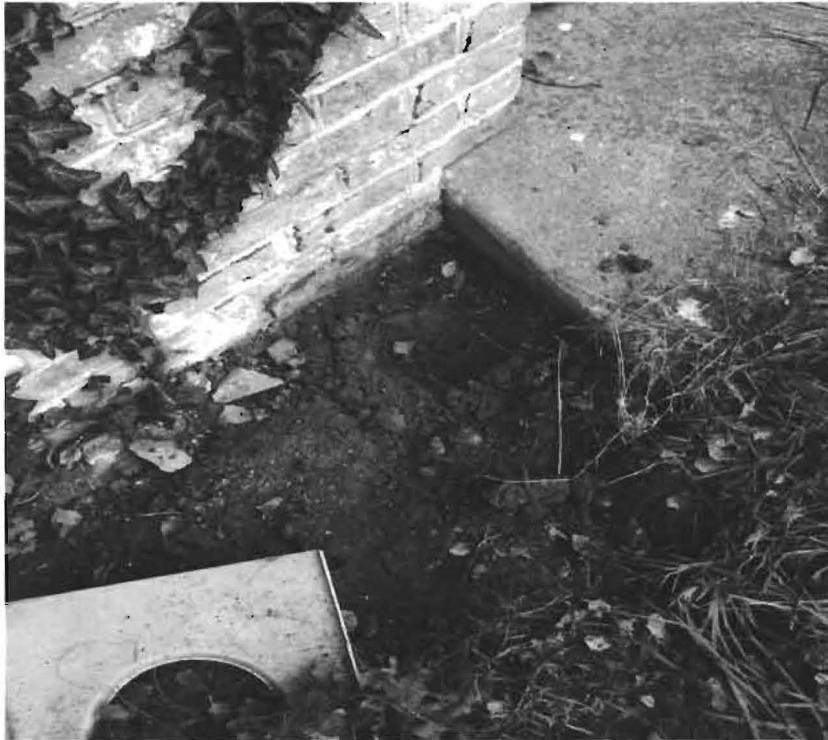
Photograph 5 Bottom of remote fill following removal
