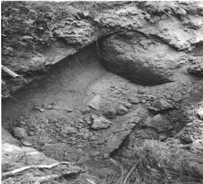
Photograph 9 Bottom of the heating oil UST excavation following removal
