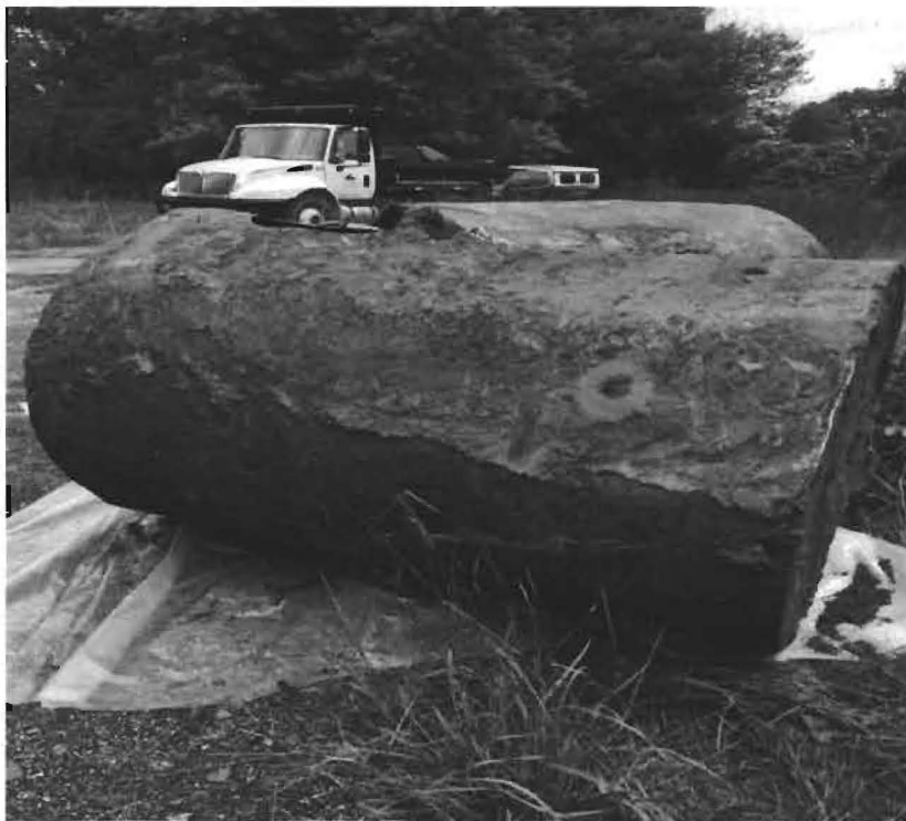
Photograph 8 Heating oil UST following removal
