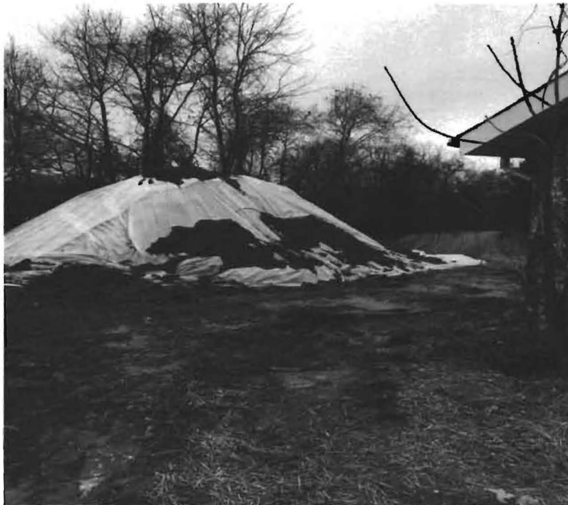
Photograph 12 Covered stockpile from soil excavation on 12-8-16
