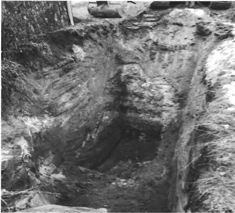
Photograph 11 Soil removal on 12-8-16
