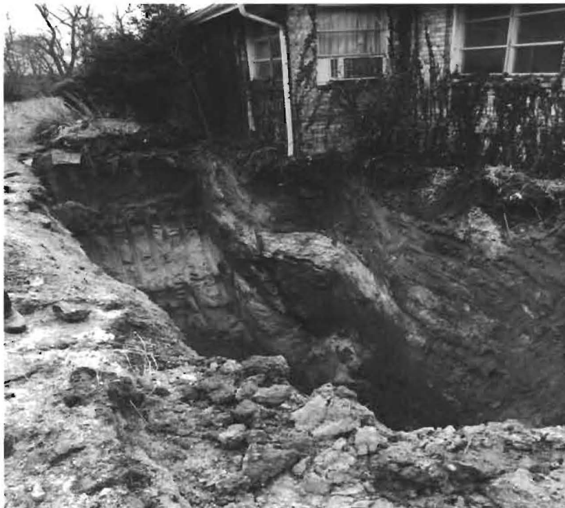
Photograph 10 Soil removal on 12-8-16
