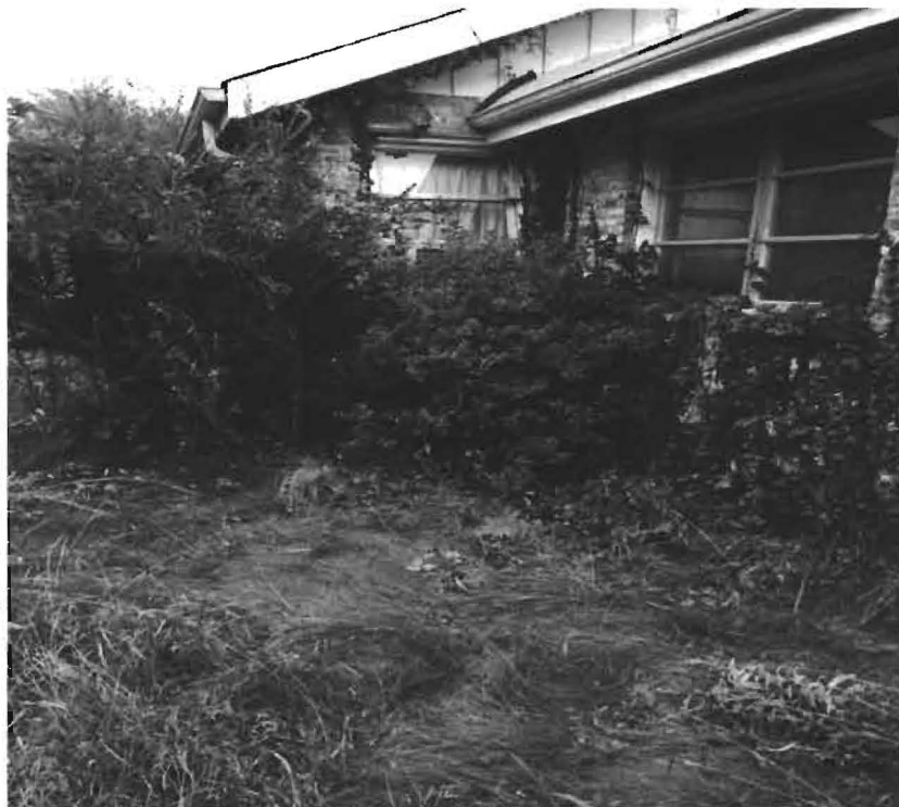
Photograph 6 Heating oil UST location on the northeastern side of the residence
