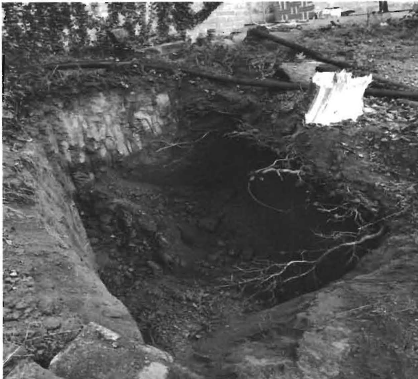
Photograph 3 Bottom of the diesel UST following removal
