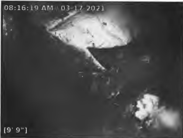
3/17/2021 8:16:19 AM Crushed portion of drainfield A.
