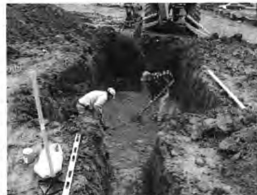
Photo 4.1.3-Bedding being spread and compacted
