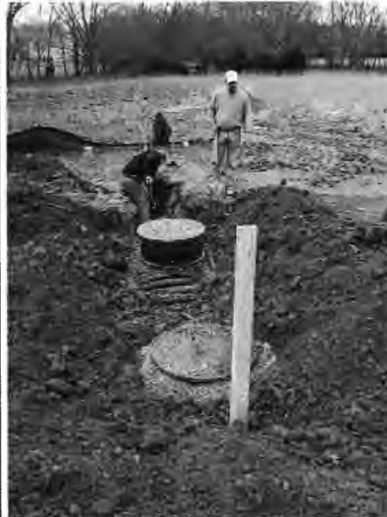
Photo 4.1.12-Example of complete backfill
