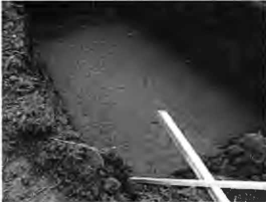
Photo 4.1.4-Bedding material prepared for setting the tank
