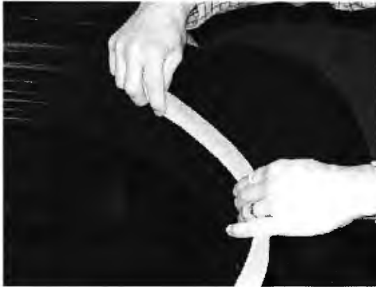
Photo 4.1.17-Applying the foam gasket
