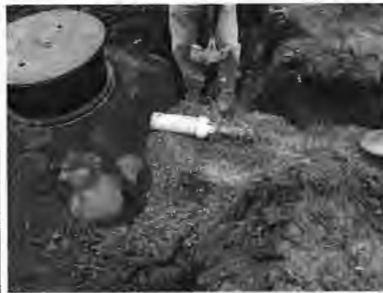
Photo 4.1.15-Example of careful and uniform backfill of piping system
