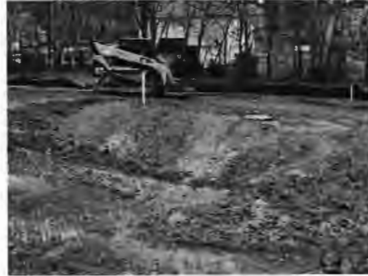
Photo 4.1.14-Example of final grading
