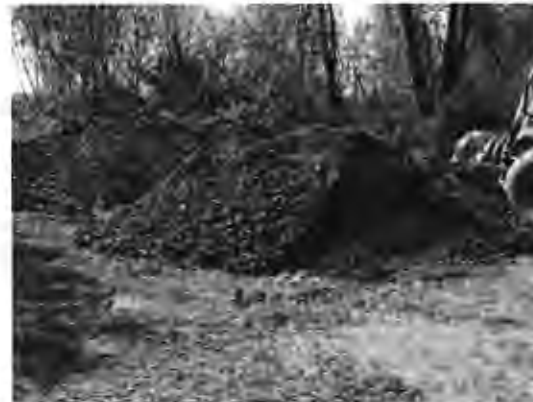
Photo 4.1.10-Example of backfilling material
