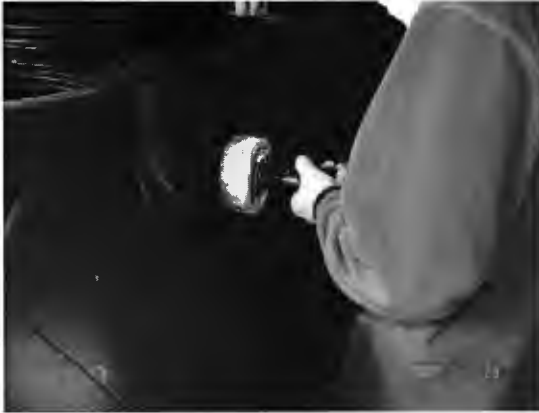
Photo 4.1.1-Drilling of inlet and outlet holes
