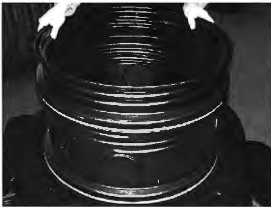
Photo 4.1.18-Riser and tank joints completely threaded in and gasketed
