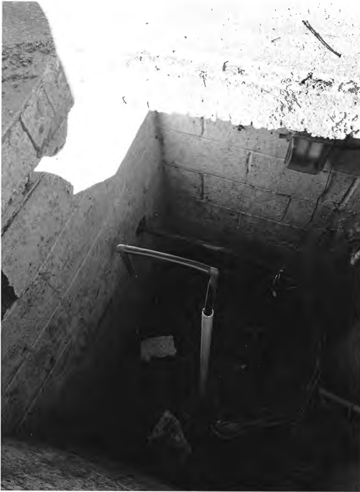
11/12/24 Well - house connection (MRS)
