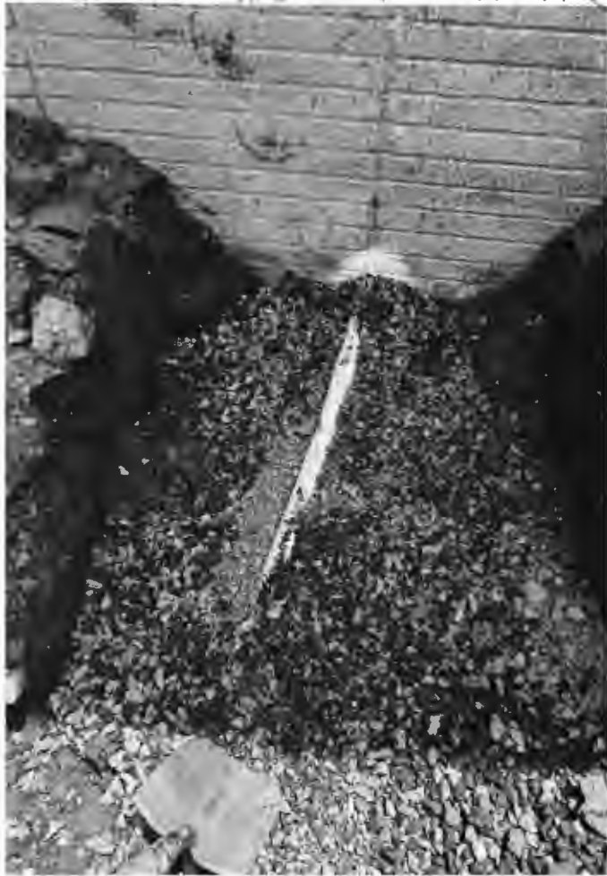
Contractor filled in over dig and sealed outside line
