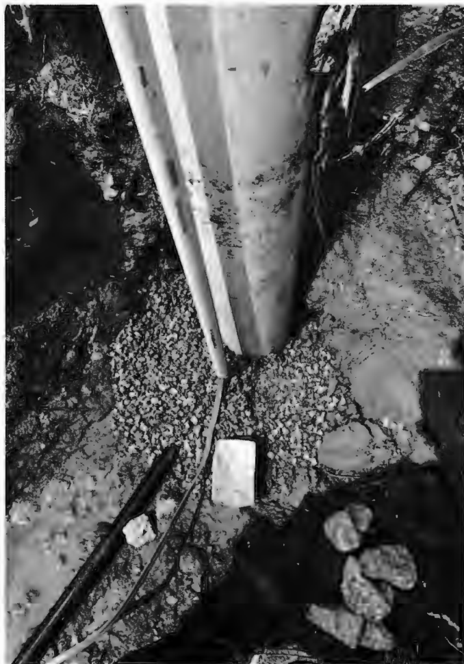
Bentonite pellets added to final 10' of annular void
