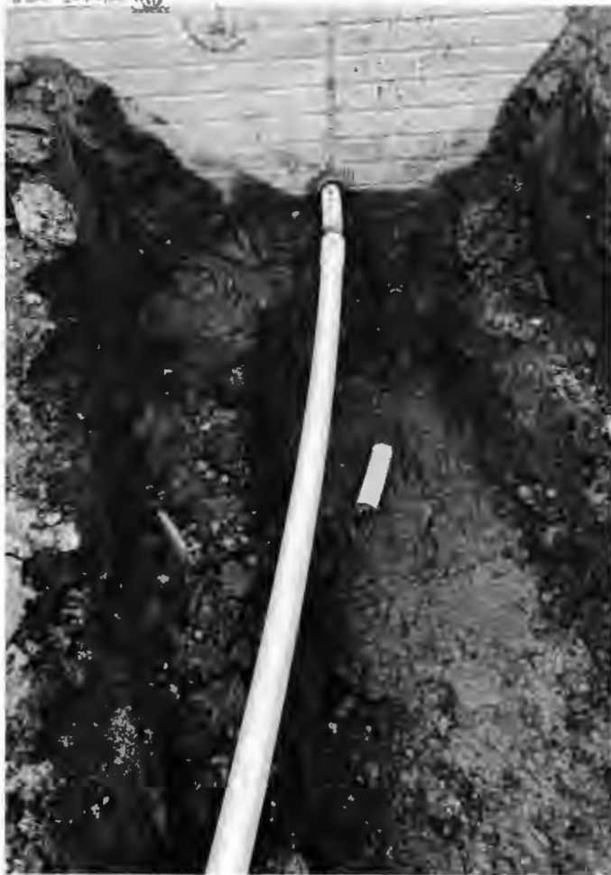
Ready to be filled and pulled in by contractor. (19)
