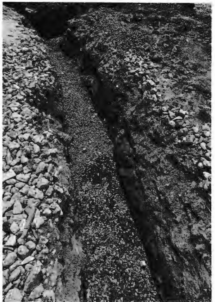
57 Stone added to well line
