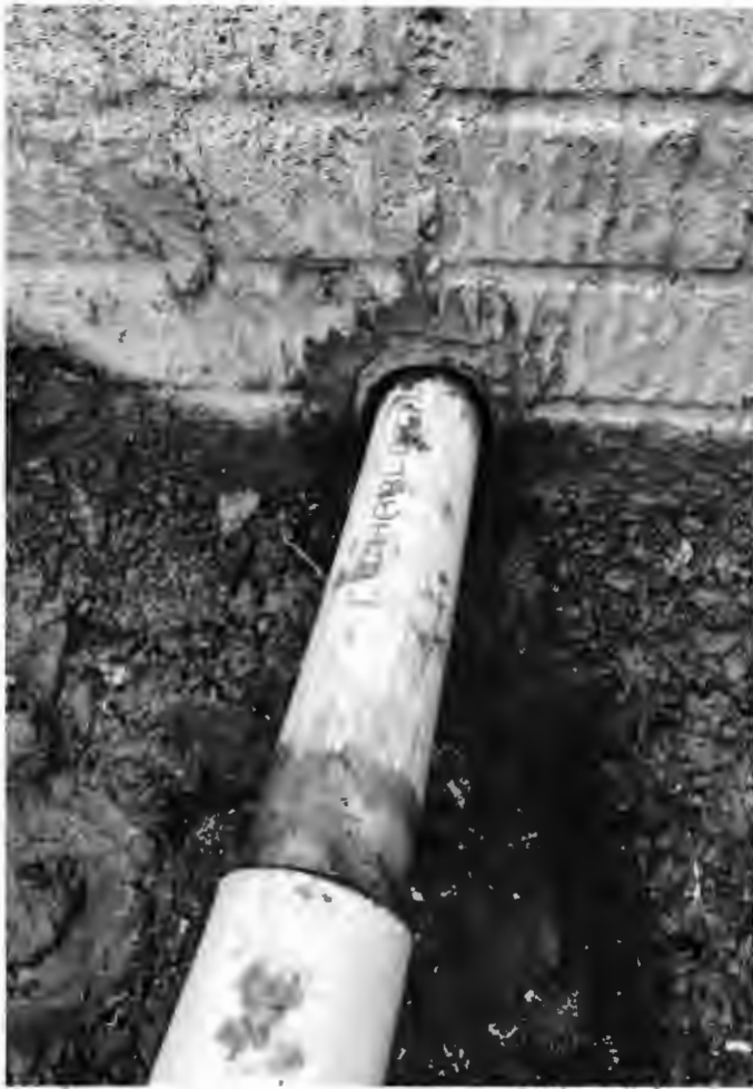
Builder has base sealed inside the house. Builder will also seal outside. (18)
