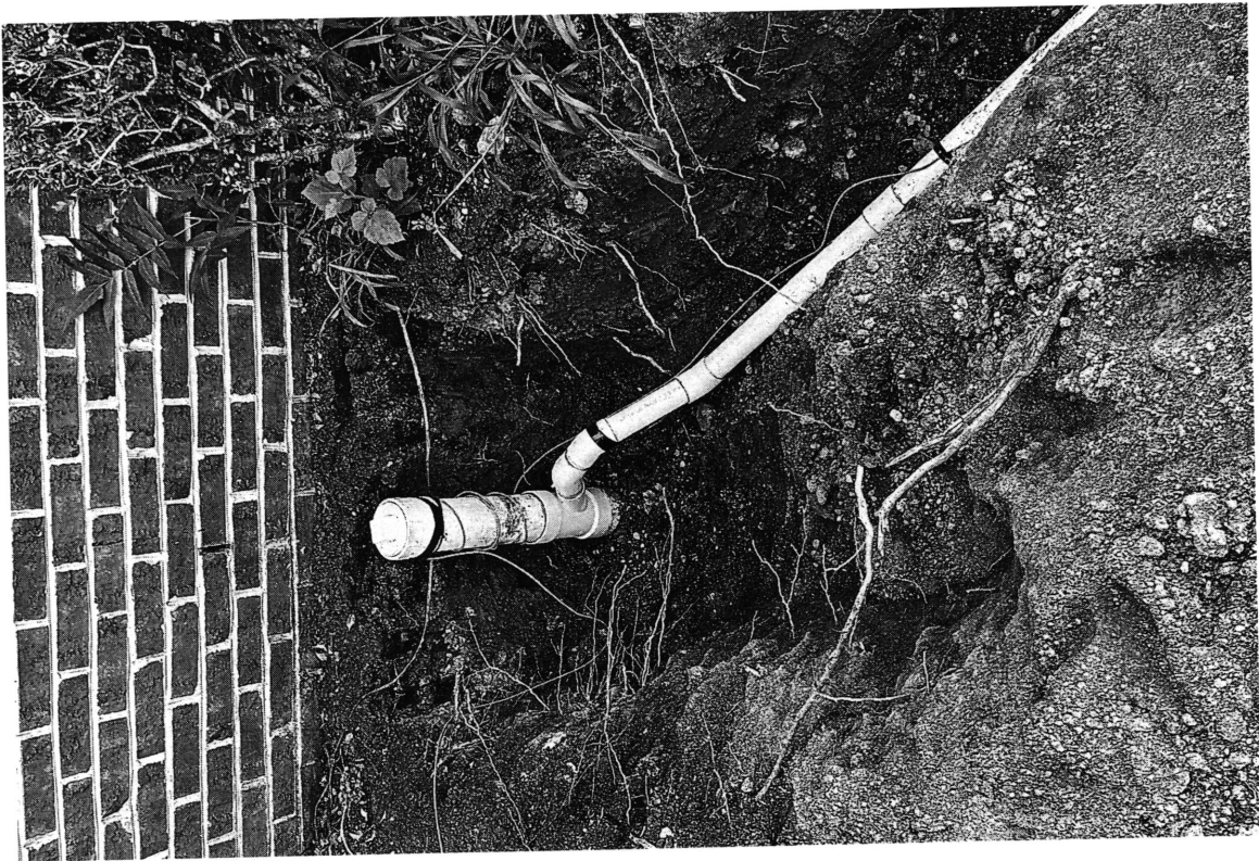
2" tie-in to existing 4" septic line (10)
