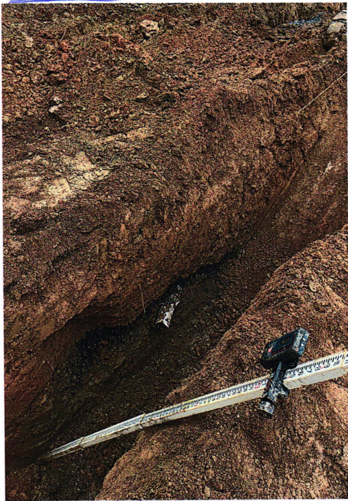
3 rd trench found while digging upper trench, ran perpendicular to trench being dug. 4' inlet. Encountered trench for about 4 feet. (MB)
