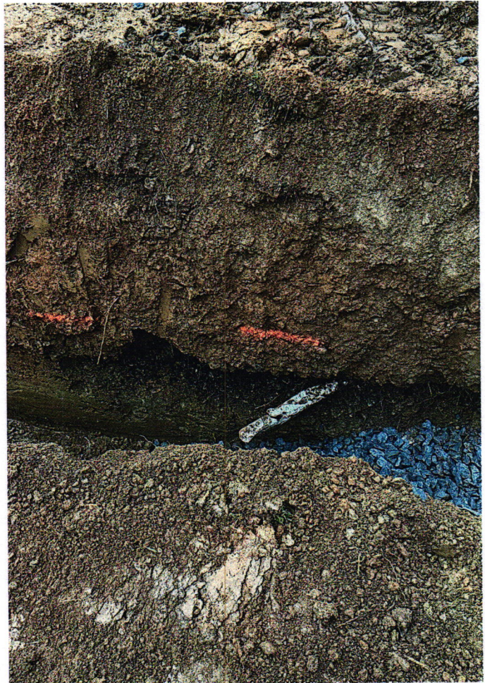
3 rd trench found while digging upper trench, ran perpendicular to trench being dug. 4' inlet. Encountered trench for about 4 feet. (MB)
