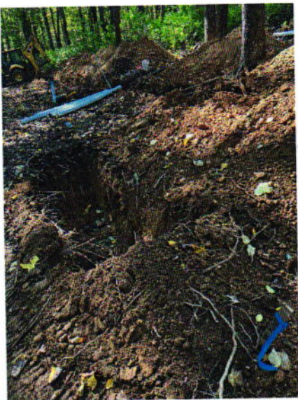
Rock @ lower left trench
