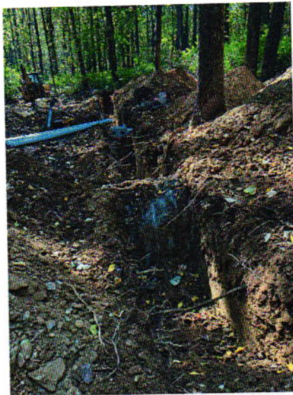
Rock @ upper left trench
