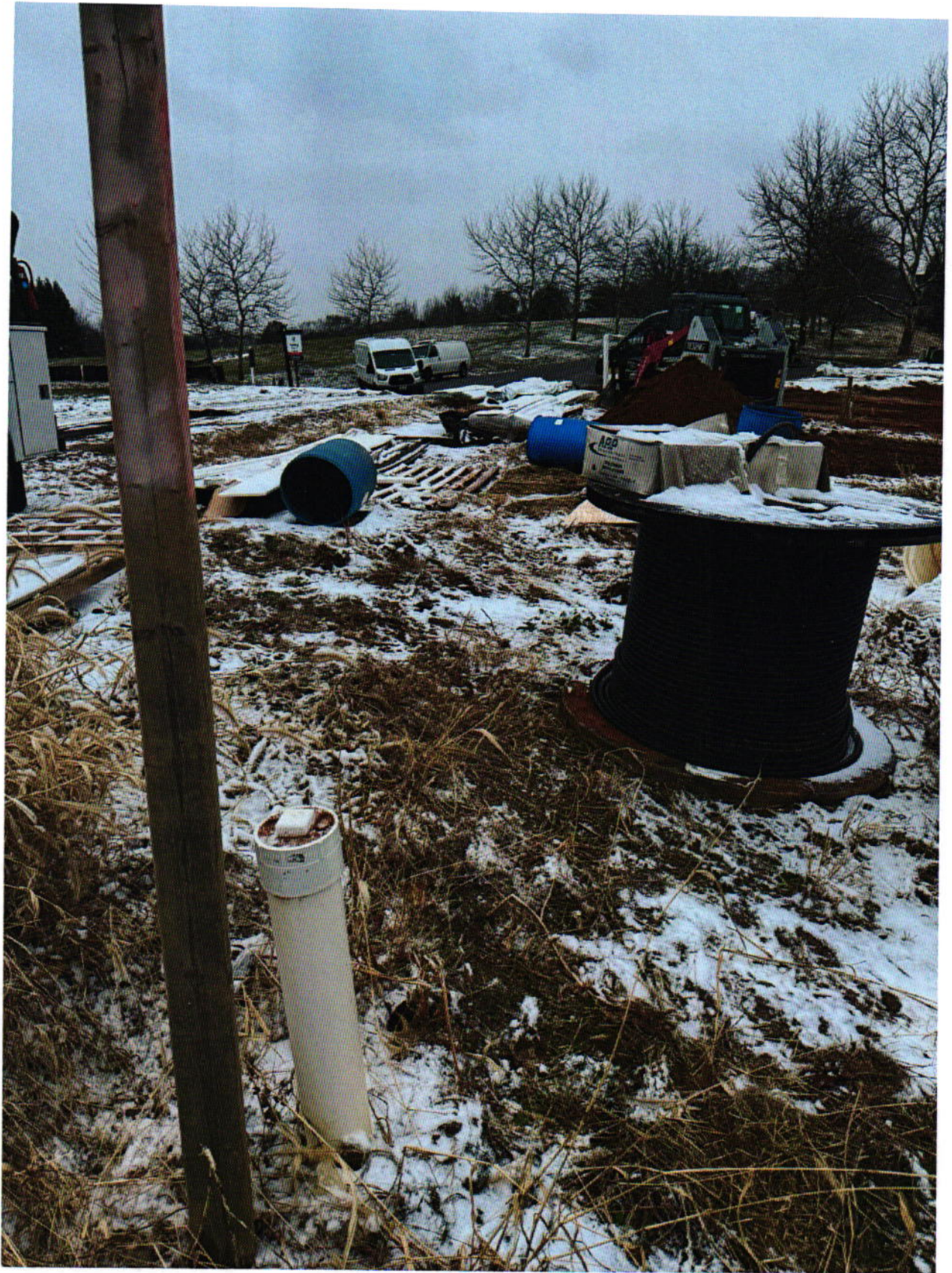
12/5/2025 - Fill & materials on upper trench. (SP)
