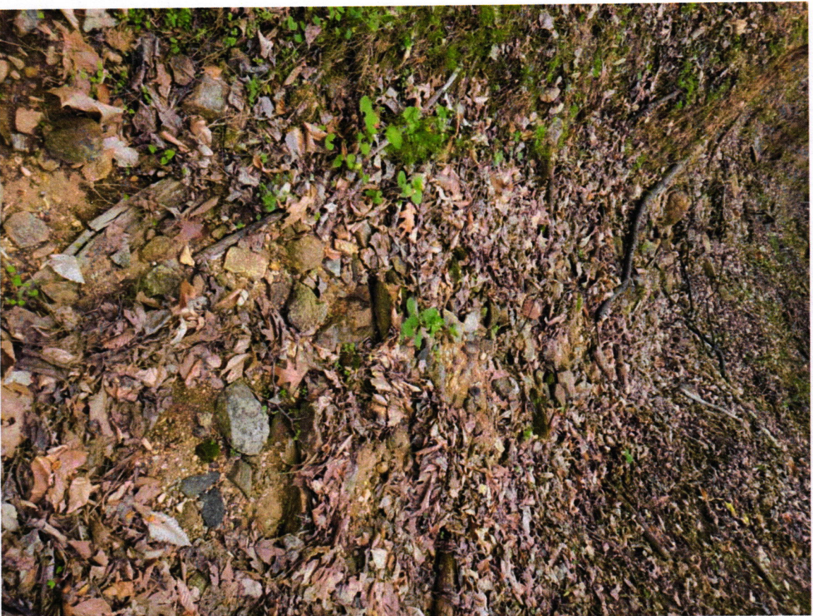
Close up of scour pattern in bottom of the drainage way. Note vegetation growing within the scour pattern
