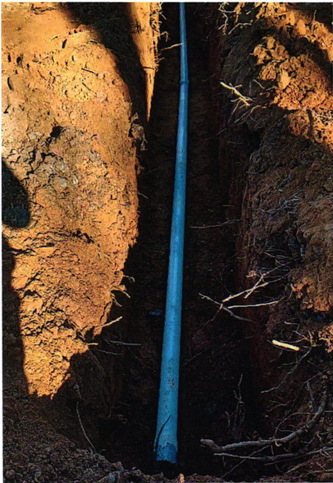
2' trench dug for FM between trench 1 & 2
