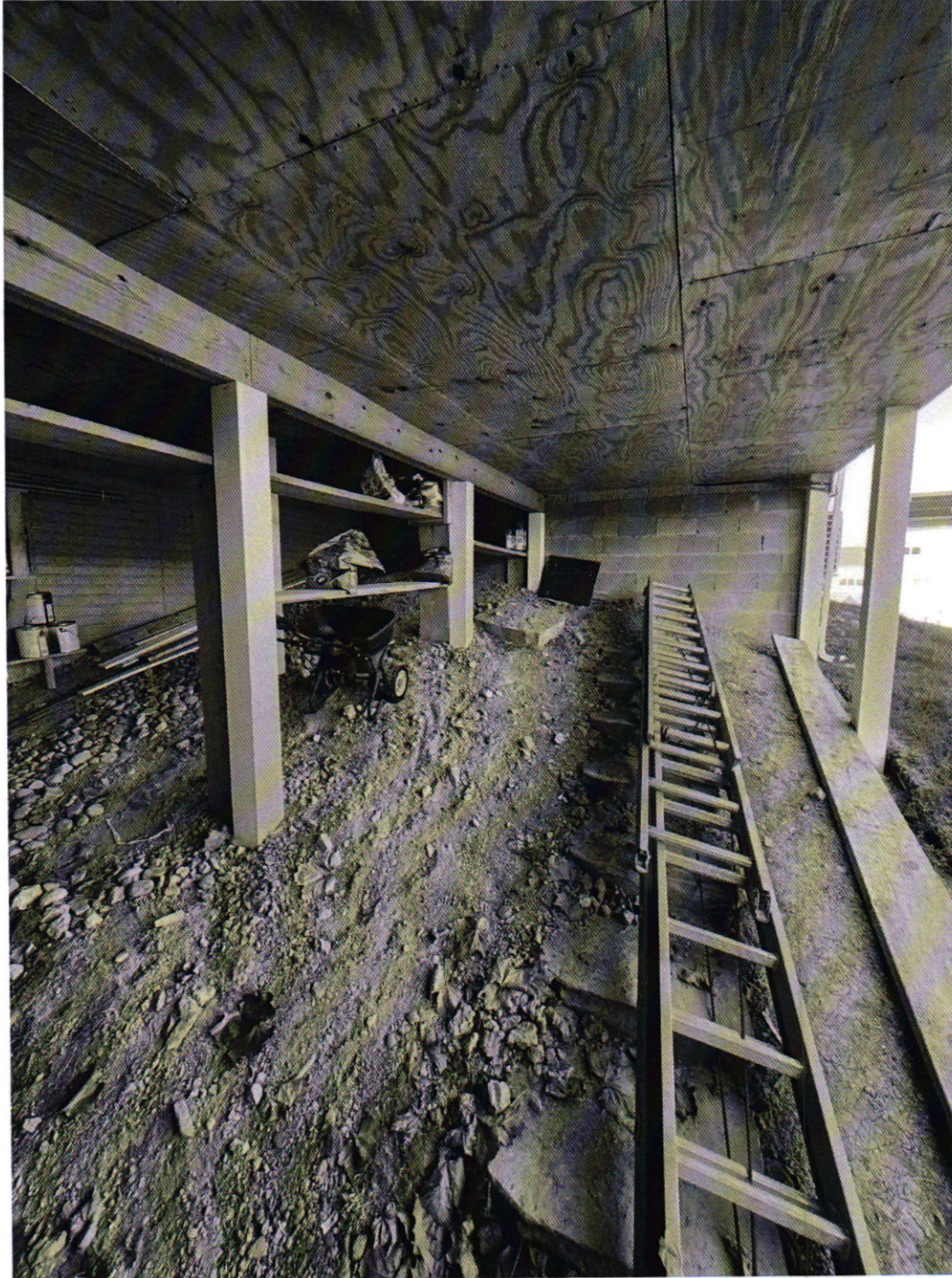
Structural support of Sunroom and void under
