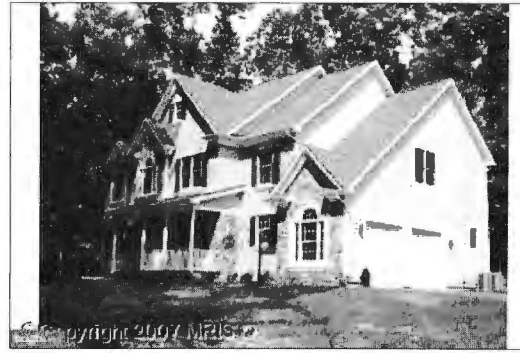
PHOTO OF EXISTING FRONT/RIGHT ELEVATION
