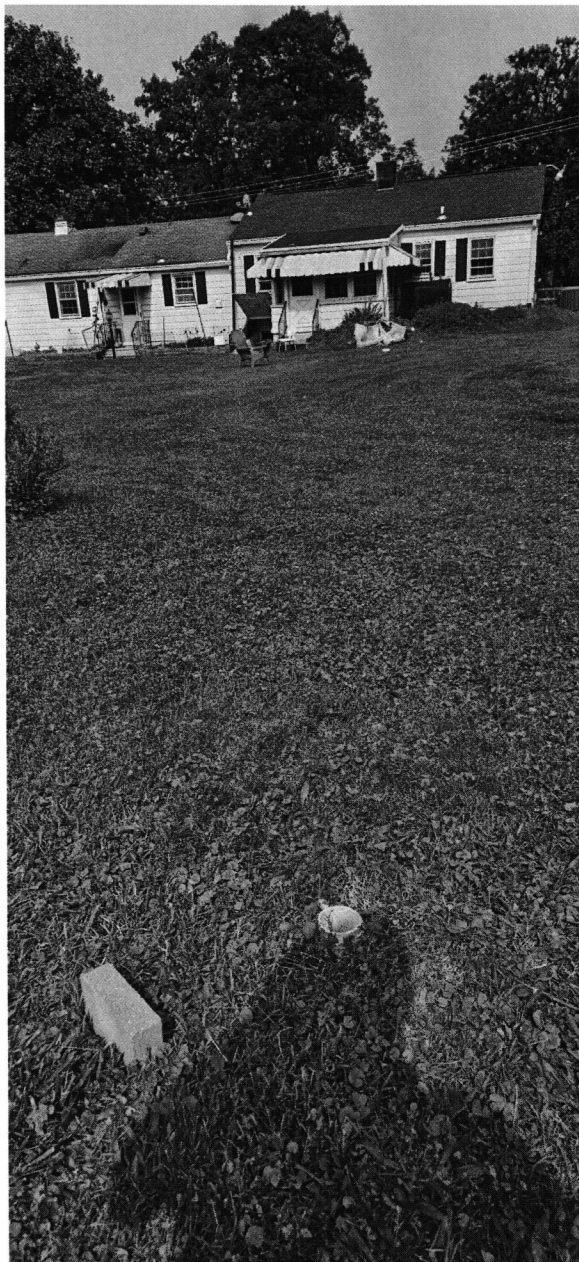
Possible c/o for drywell
