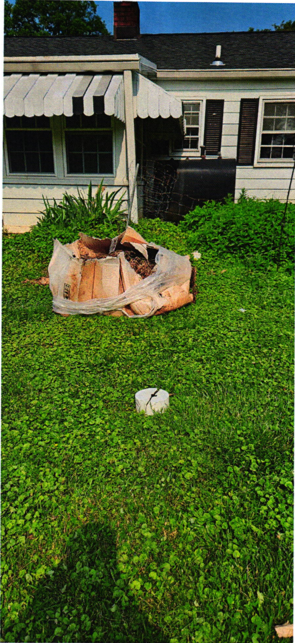
Septic Tank c/o
