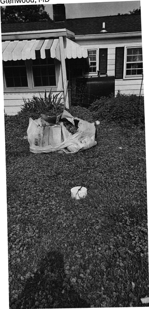
Septic Tank c/o
