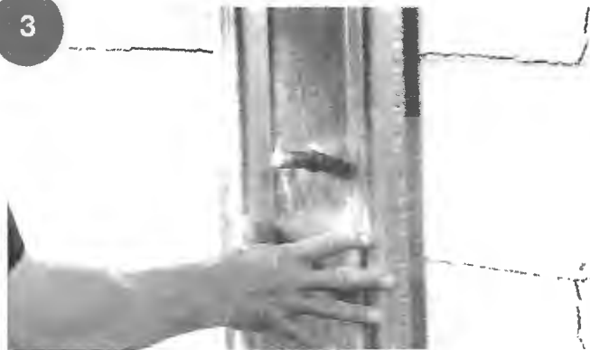
3 Install wall anchor plate.
