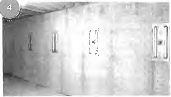
4 Replace soil and sod. Tighten wall anchor to specified torque rating.
