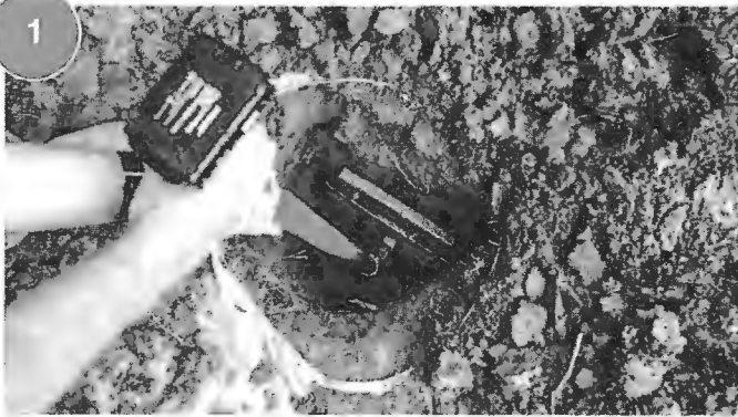
1 Carefully remove sod away from foundation wall, excavate hole several feet deep and insert earth anchor plate.
