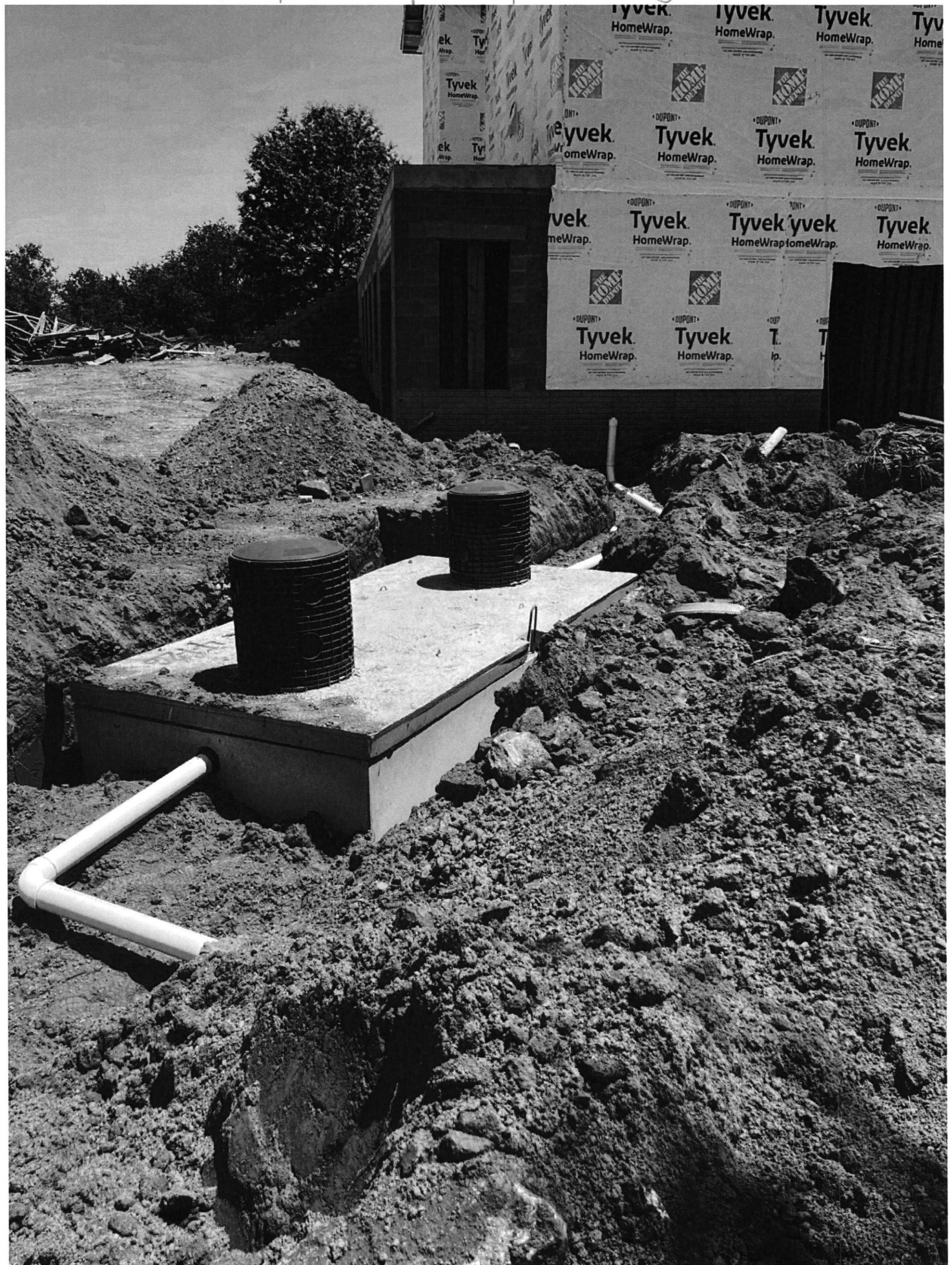
1210 Sugar Maple Drive - Septic tank replacement install
