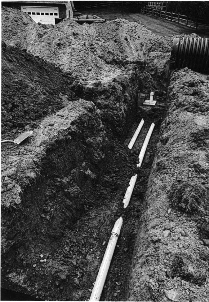
D-box and back line installation
