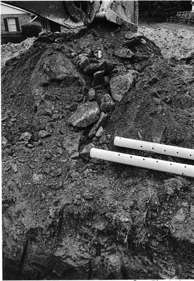
Rock encountered on trench 3 from 7' to 16' lengthwise
