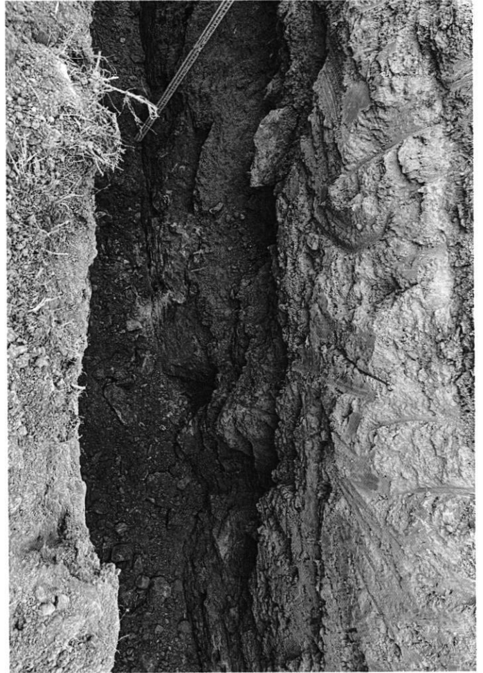
Rock encountered on trench 3 had a depth of 3' to 10'
