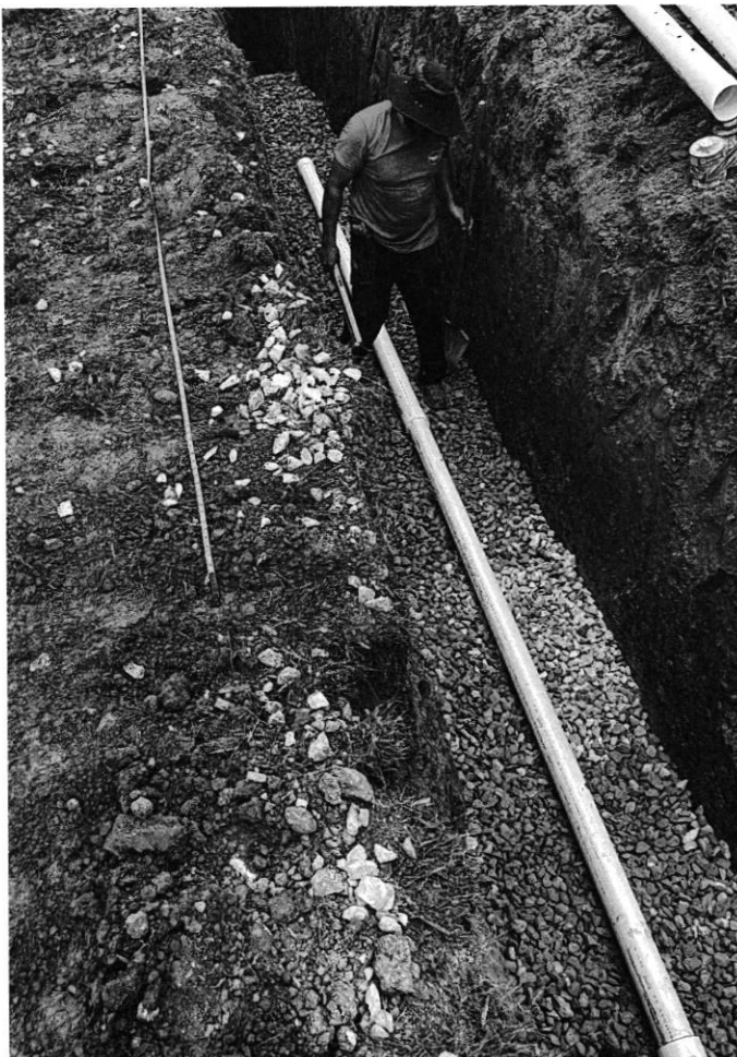
Contractor added solid pipe from 7' to 16'
