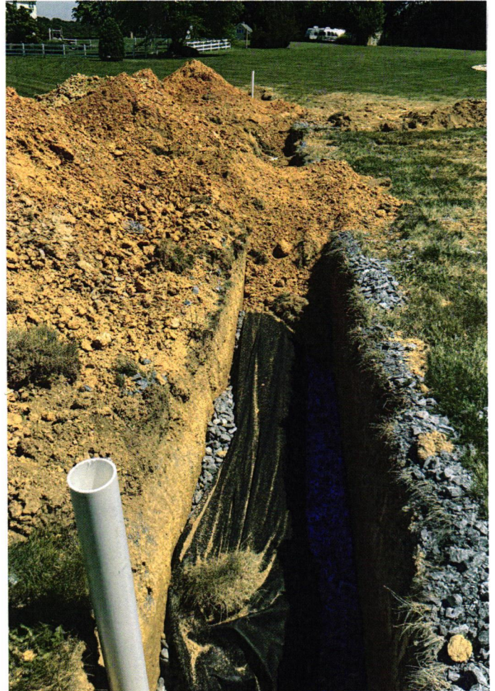
Bottom two trenches
