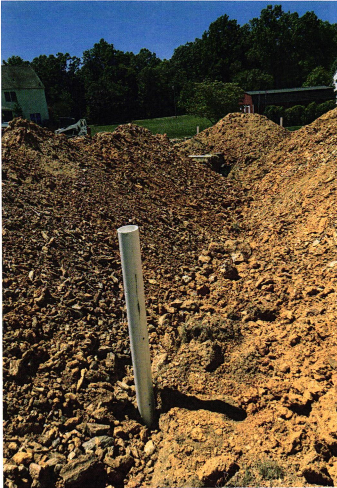
Middle trench covered
