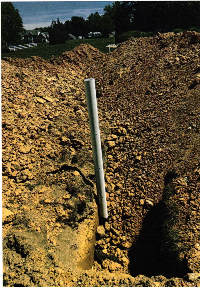
Middle trench covered
