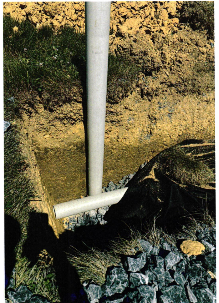
Bottom trench pipe on side of trench
