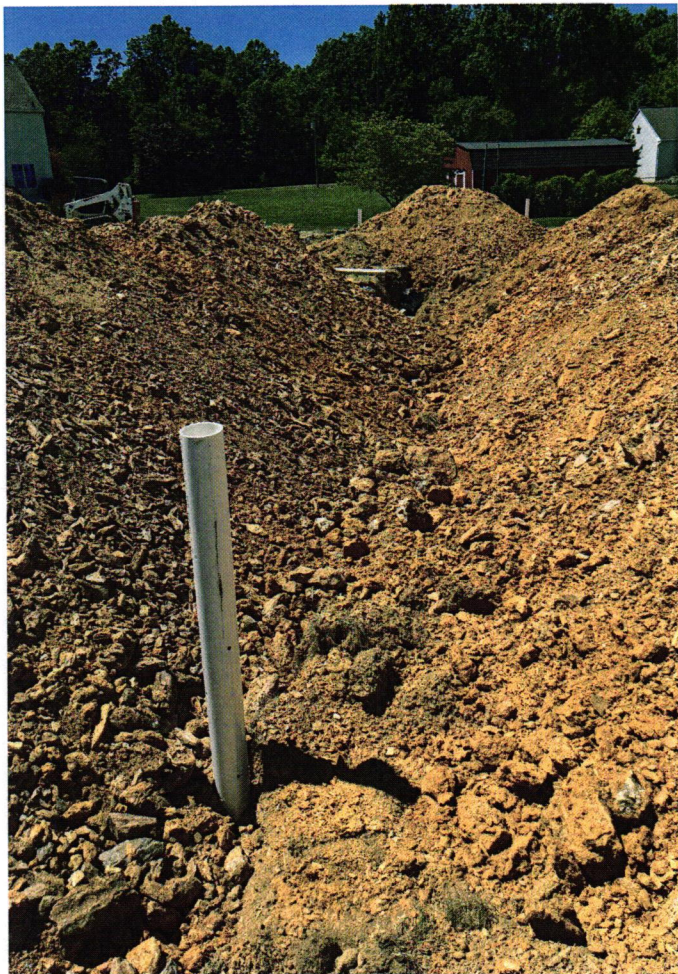
Middle trench covered
