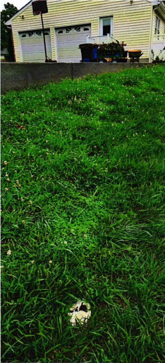
Septic Tank Cleanout
