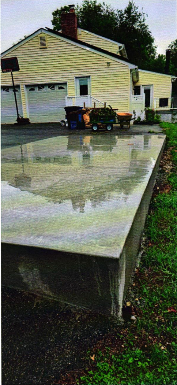
Slab for proposed shed
