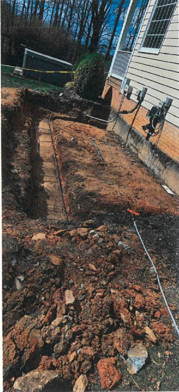
Addition Foundation Started
