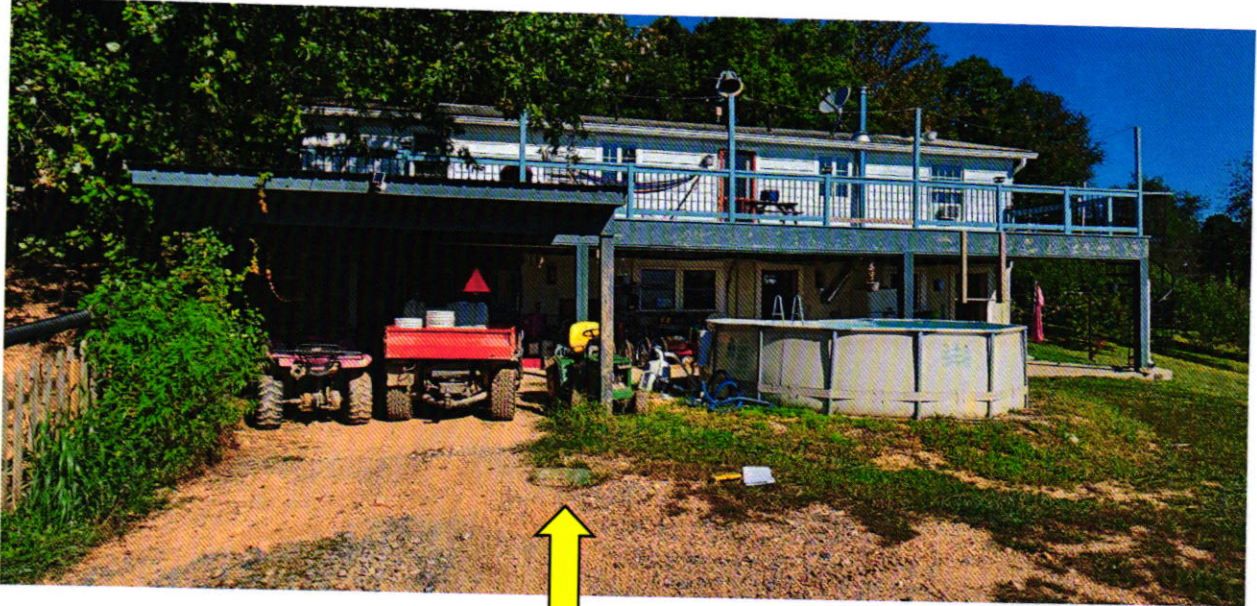
Septic tank manhole cover.
