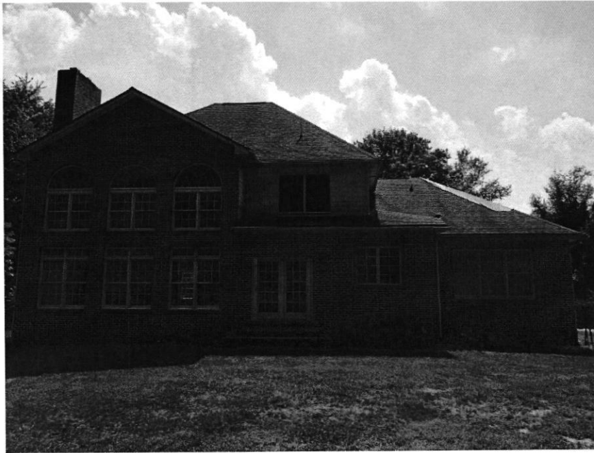
Photograph 3 - View of the rear elevation of the subject property.
