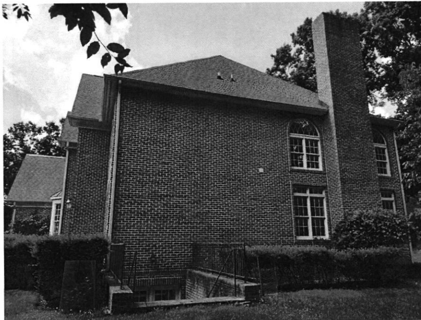
Photograph 4 - View of the right elevation of the subject property.
