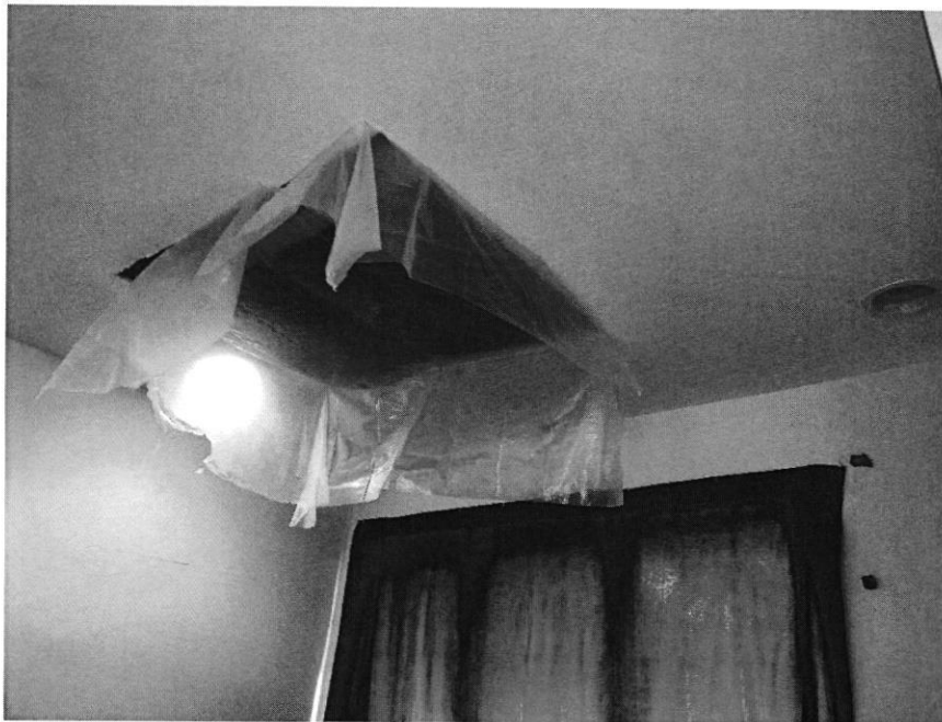
Photograph 14 - View of access hole cut in left-side bathroom ceiling.
